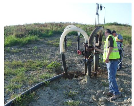
*Underground surface trenches and gas wells capture odorous gases and route to a flare to be destroyed*
